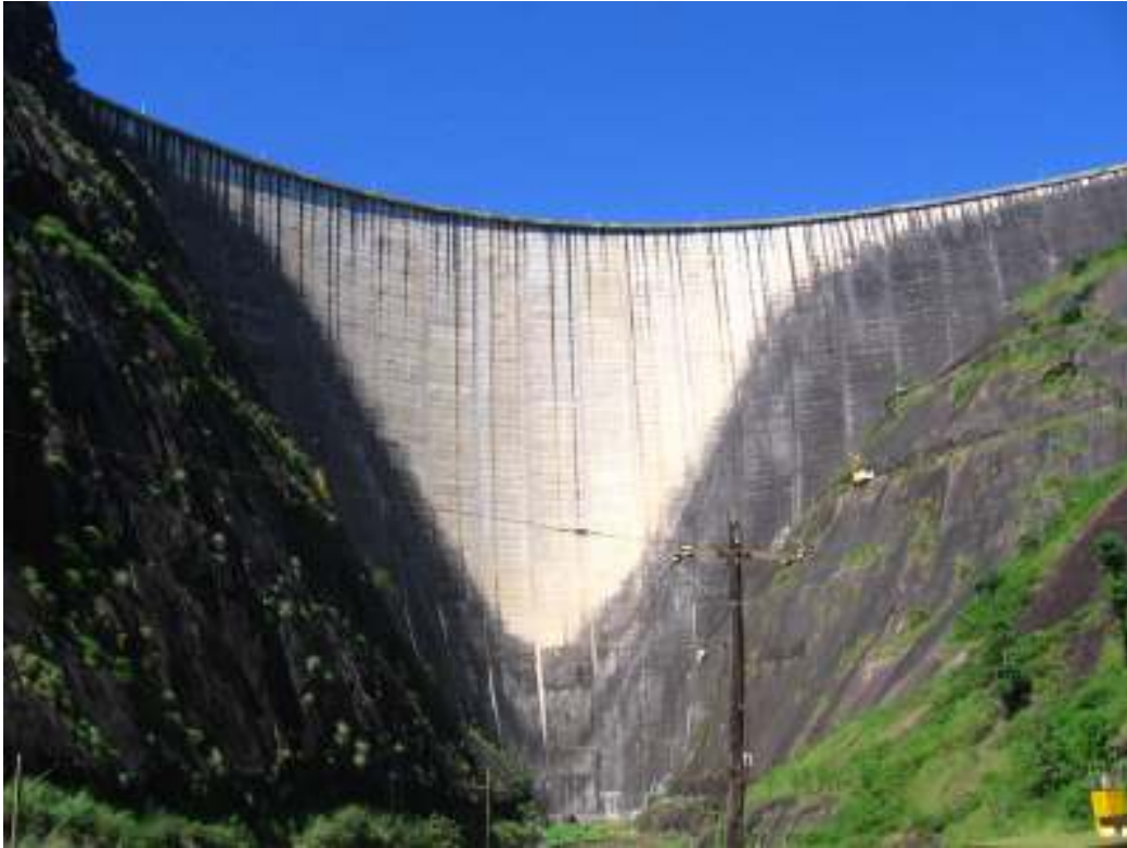
IDUKKI ARCH DAM
